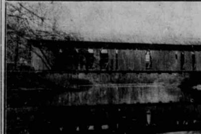
White's bridge, only covered bridge in Ionia county, is an historic landmark in Keene township. It was constructed in 1867 of hand-hewn timber. At present it is condemned for vehicles weighing more than two tons. Note the striking reflection of the structure in the waters of the Flat river.
